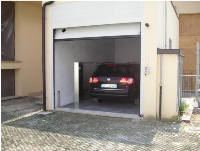
Sectional door application on the courtyard floor
