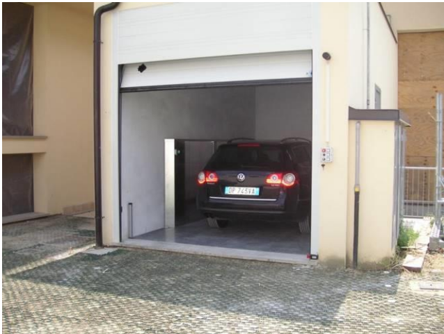
Sectional door on courtyard level
